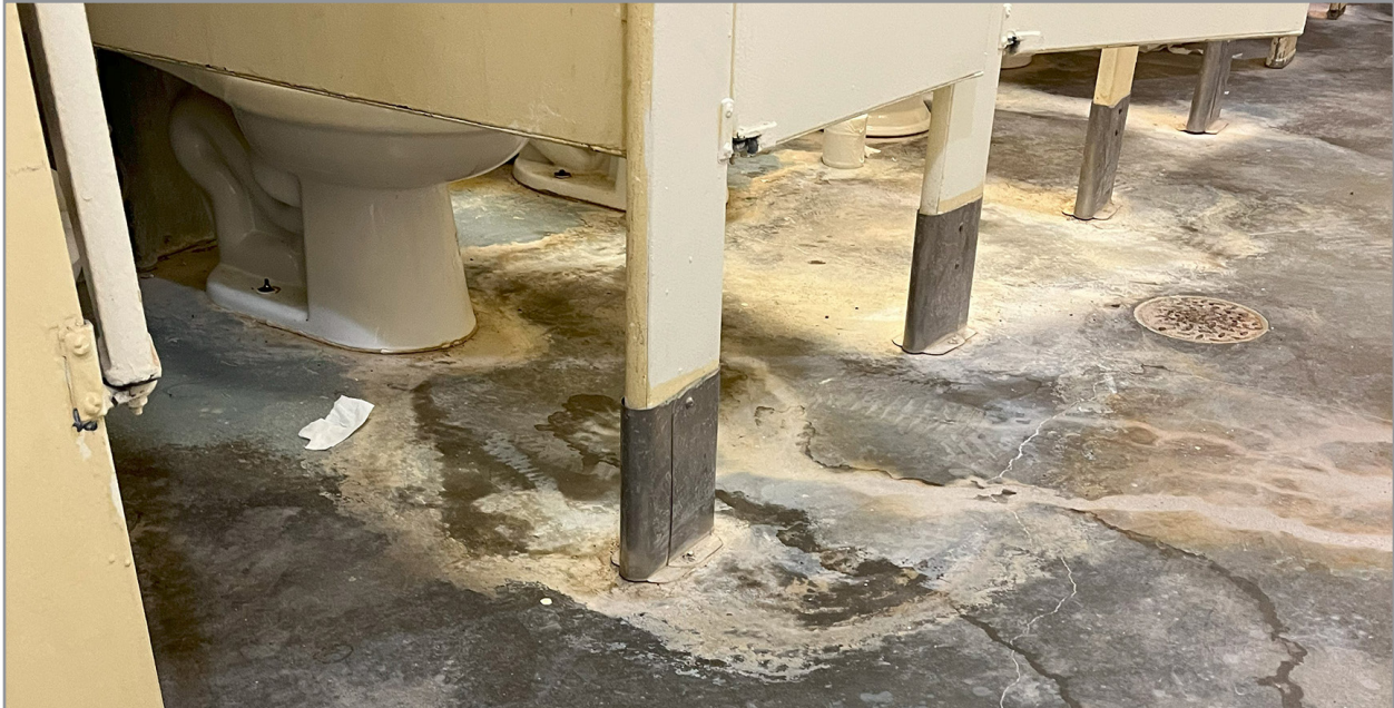
Figure. The Doña Ana Range Complex Bathroom with Sewage Leaking from the Plumbing Source: The DoD OIG.
