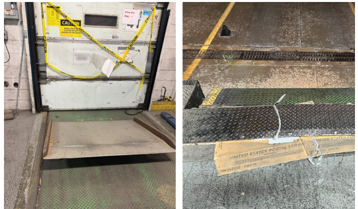
Figure 3. Inoperable Door and Dock Plate
