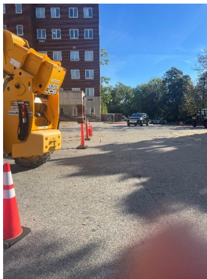
Figure C.2. Photo of drive-up ramp to clinic entrance.
