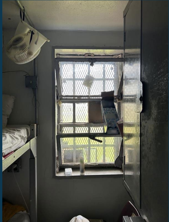
Left, Housing Unit Bathroom Window with a Missing Pane, Rusting Edges, and Exposed Masonry at the Edge of the Frame, Right, Cell Windowpane Covered with Cardboard and a Towel Stuffed in the Top Right of the Window Frame
