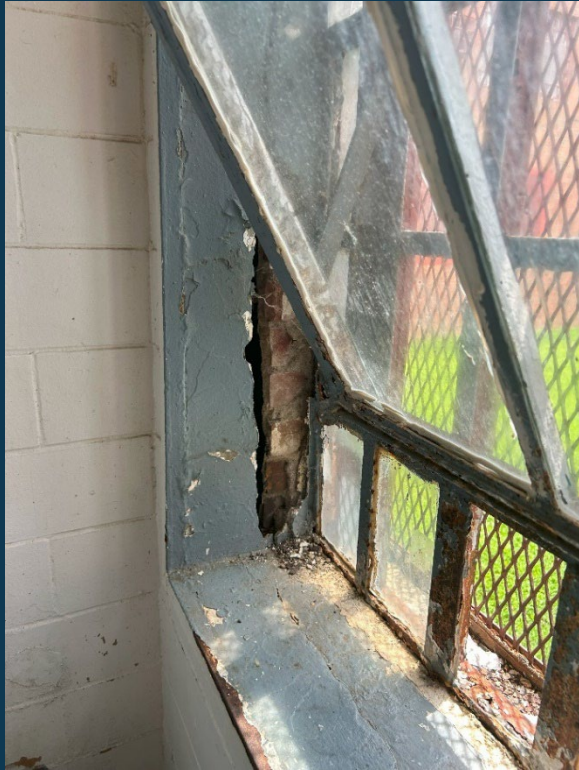
Left, Housing Unit Bathroom Window with a Missing Pane, Rusting Edges, and Exposed Masonry at the Edge of the Frame, Right, Cell Windowpane Covered with Cardboard and a Towel Stuffed in the Top Right of the Window Frame
