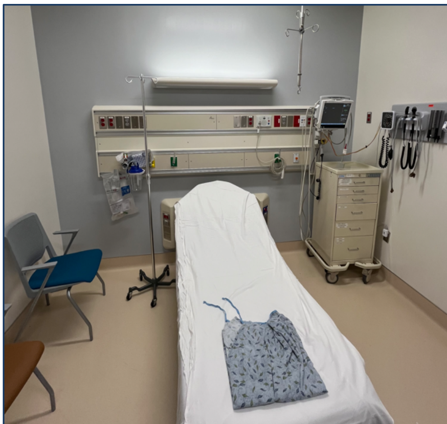
Figure 3. An exam room added to the Audie L. Murphy emergency department in phase 3 has a headwall containing medical air, oxygen, and vacuum lines.
