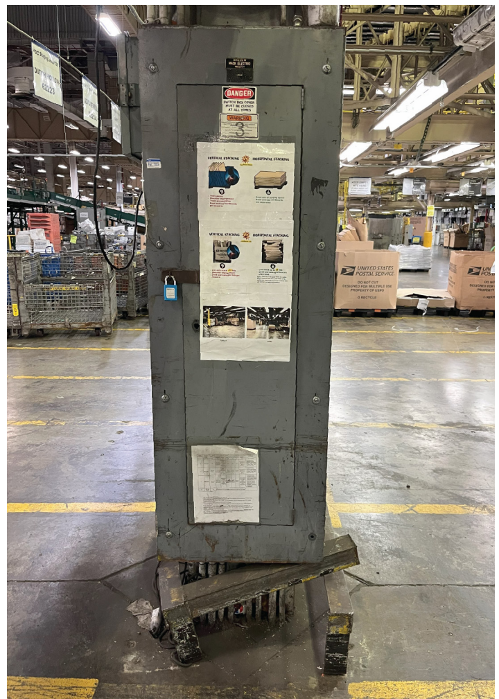
Figure 7. Damaged and Unstable Electrical Panel Base
