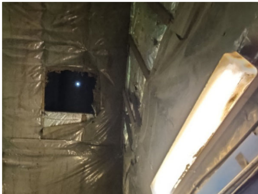
Figures 7a. Hole in the solid waste barn ceiling; 7b. Solid waste barn lighting
