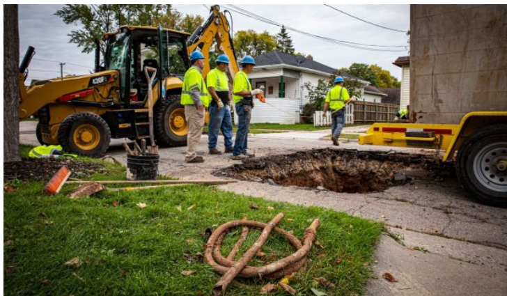
Utility employees working on a lead service line. (EPA image)
