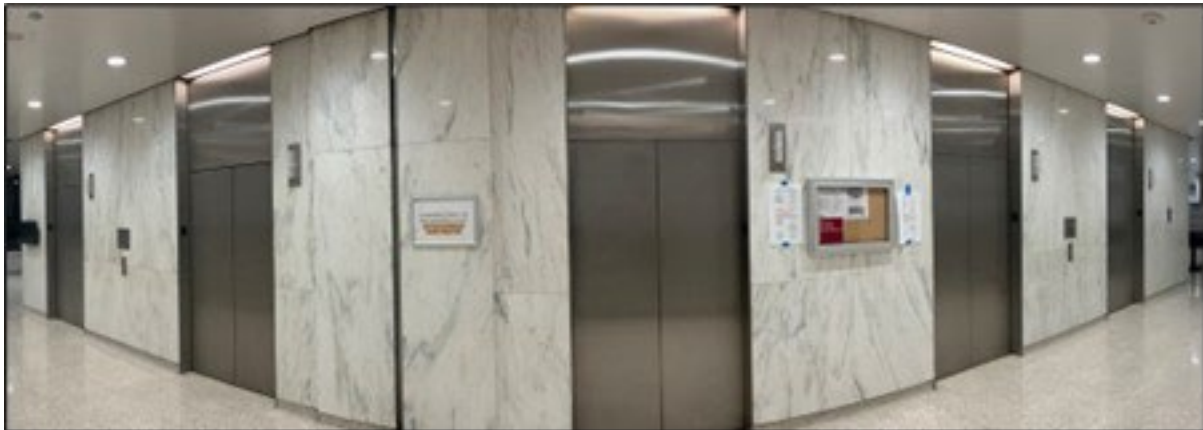
Figure 5. Elevator Lobby Without the Required Evacuation Route Diagram 13
