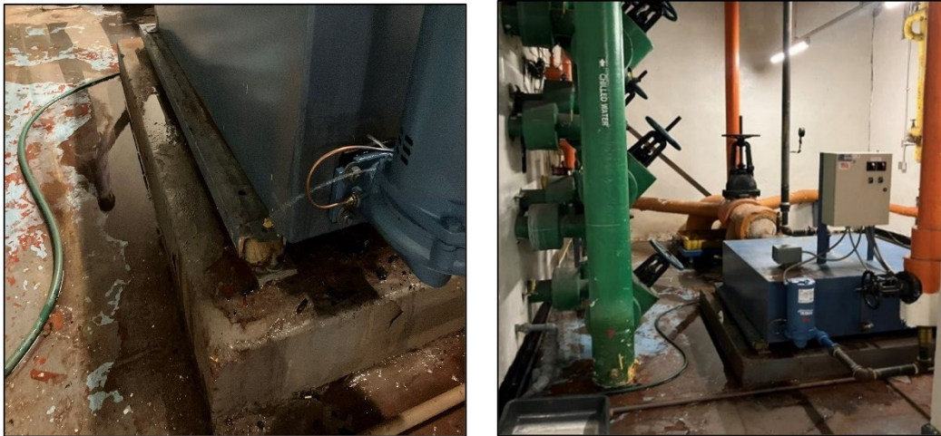
Figure 7. Leaking Condensate Pump with No Precautionary Signage 17
