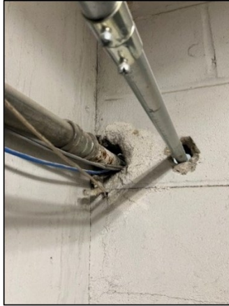
Figure 3. Examples of Gaps in the Fire-Resistant Walls of an Elevator Machine Room 11
