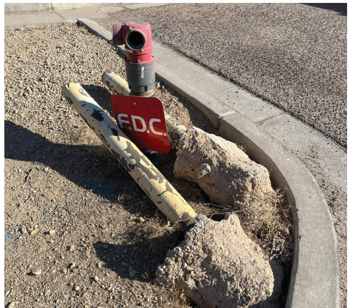
Figure 7. Damaged Protective Pylons at the Mesa Four Peaks Station
