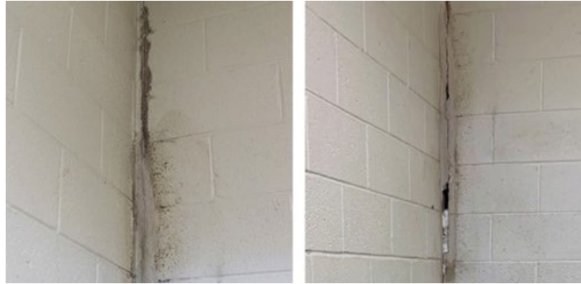
A crack in the wall between adult and juvenile holding cells observed in 2015 (left) and 2022 (right). This crack prevents sight and sound separation between adult and juvenile holding areas, which is a requirement under national standards adopted pursuant to the Prison Rape Elimination Act. Source: OIG.
