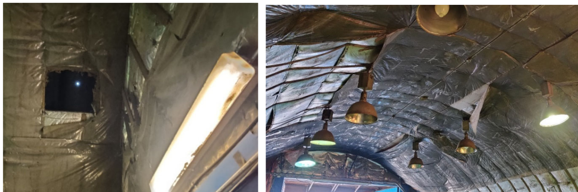
Figures 7a. Hole in the solid waste barn ceiling; 7b. Solid waste barn lighting
