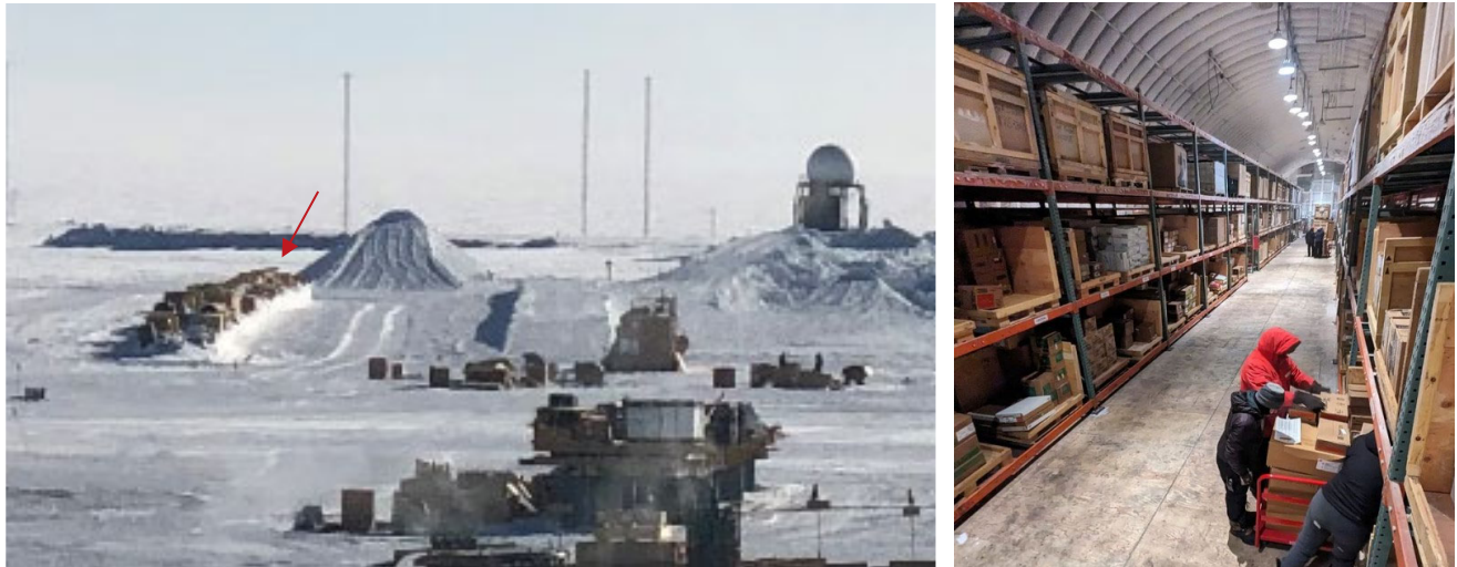
Figure 12a. South Pole Station snow berm storage; 12b. Underground logistical arch storage
