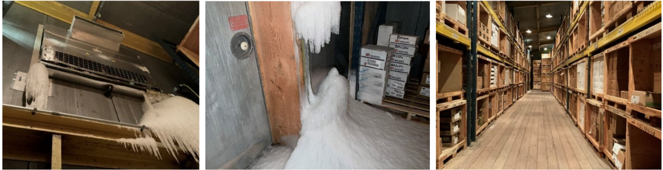
Figure 4a. Leaking condenser; 4b Ice fall; 4c. Frozen Food Warehouse at McMurdo
