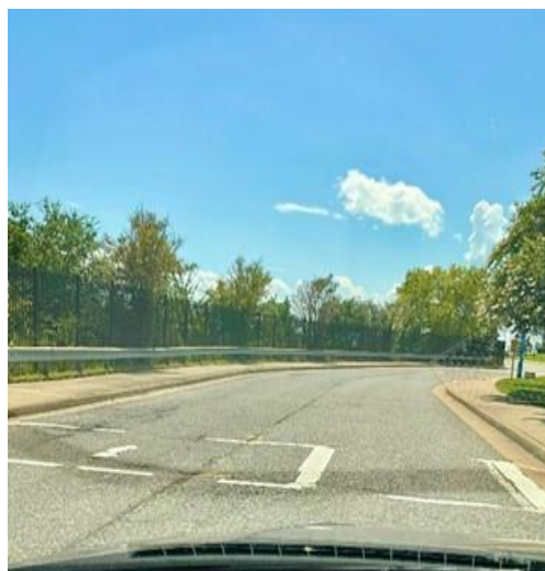
Figure C.2. Photo of an example of faded markings at one of the facility's crosswalks. Source: Photo taken by an OIG inspector.
