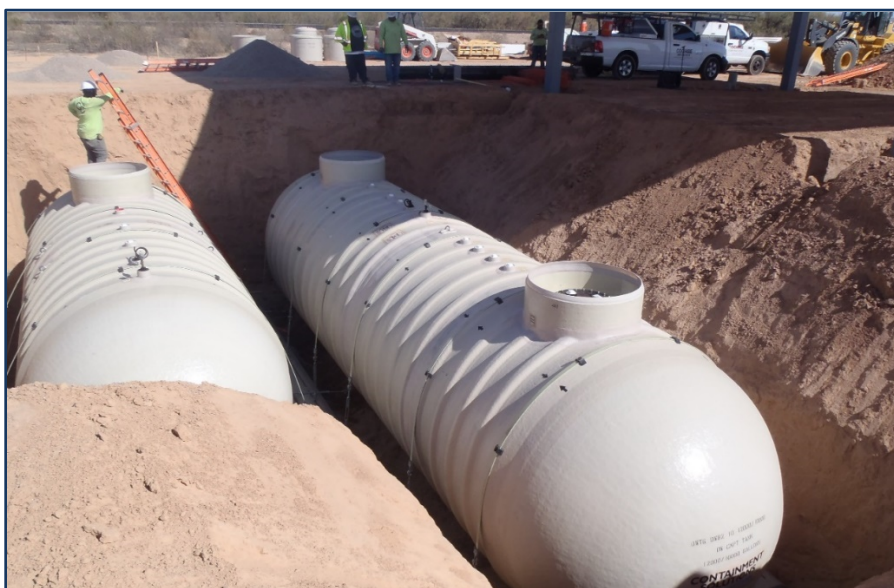
Figure 1. Two new storage tanks being installed.
