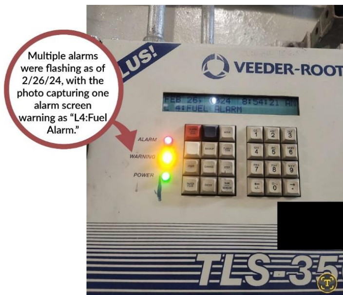
Figure 4. The Tibor Rubin VA Medical Center's Veeder-Root TLS-350 system console shows a status bar display with active alarms and warnings. The alarm displayed in the photo could indicate fuel vapor or liquid has been detected. Source: VA OIG, February 26, 2024.
