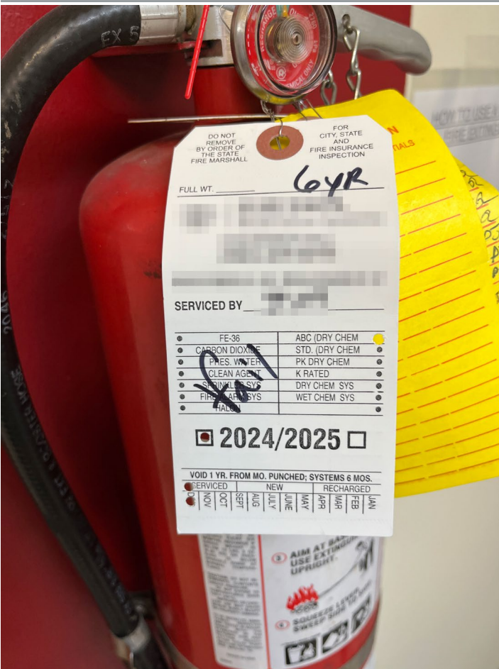
Figure 4. Failed Annual Inspection
