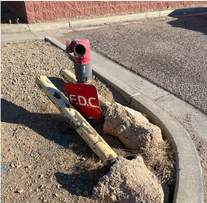
Figure 5. Damaged Protective Pylons
