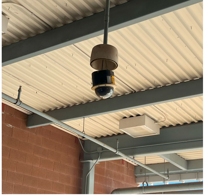
Figure 6. Damaged Security Camera
