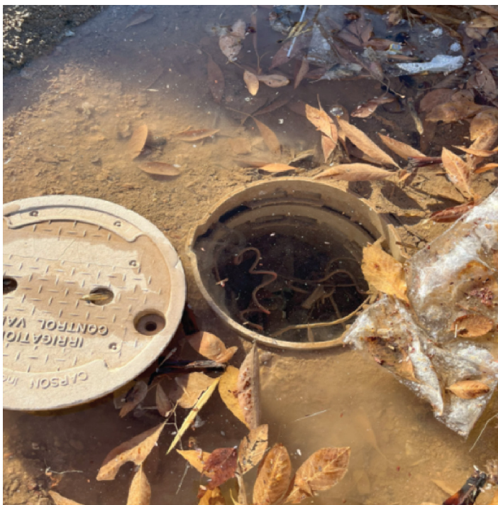
Figure 3. Irrigation System Water Leak
