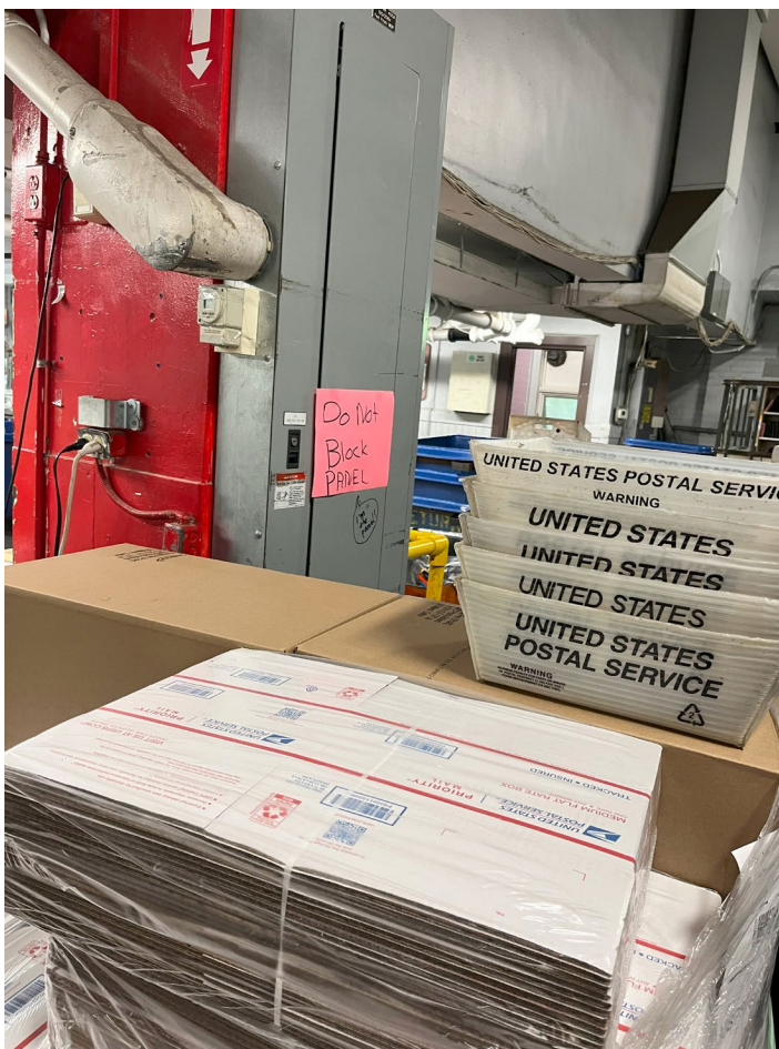
Figure 5. Example of a Blocked Electrical Panel in the Brookline Branch Workroom Area
