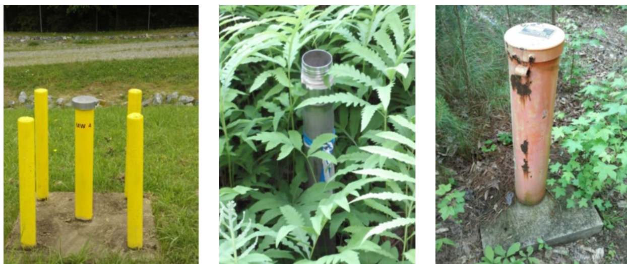
Figure 6: Examples of groundwater monitoring wells
