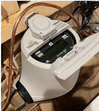
Source: EPA OIG image of a water meter.
