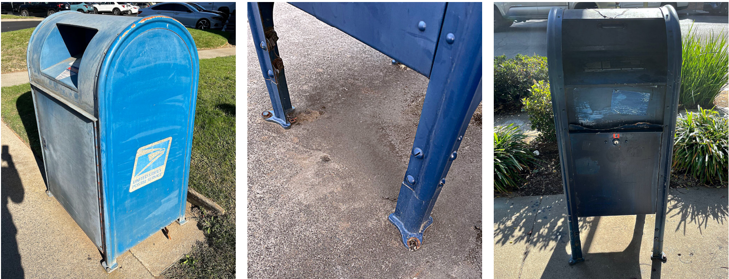
Figure 7. Sacramento, CA, Blue Collection Boxes With Corrosion, Missing Bolts, and Door Gap
