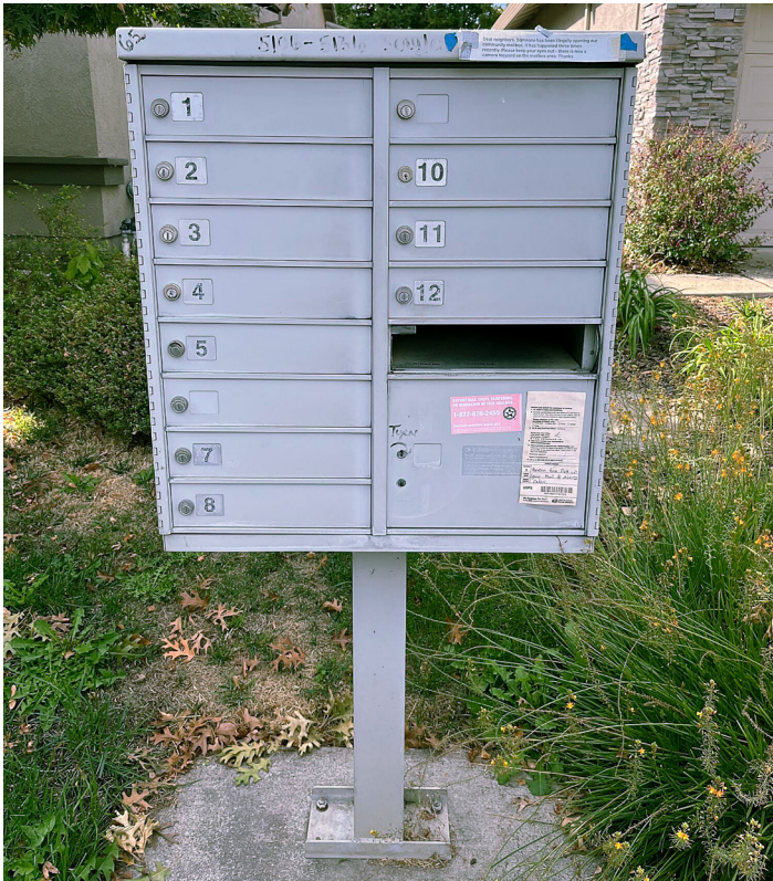
Figure 8. Sacramento, CA, Cluster Box Unit With Door Gap/Missing Door
