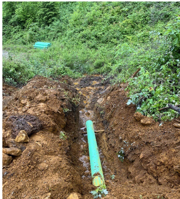
Figure 4. Drainage pipe installed on the Daniel Boone National Forest to reroute acidic mine drainage. The installation was funded through IIJA. Photo by FS.
