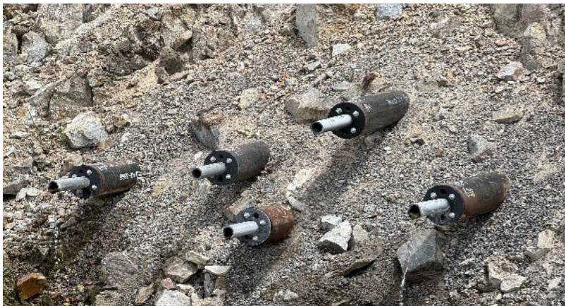
Figures 2 and 3. The Beal Mountain open-pit mine is the site of multiple projects funded by IJJA. Horizontal drains were installed to reduce groundwater infiltration of the leach pad at the Beal Mountain mine. Project funded by IJJA. Photos by OIG.
