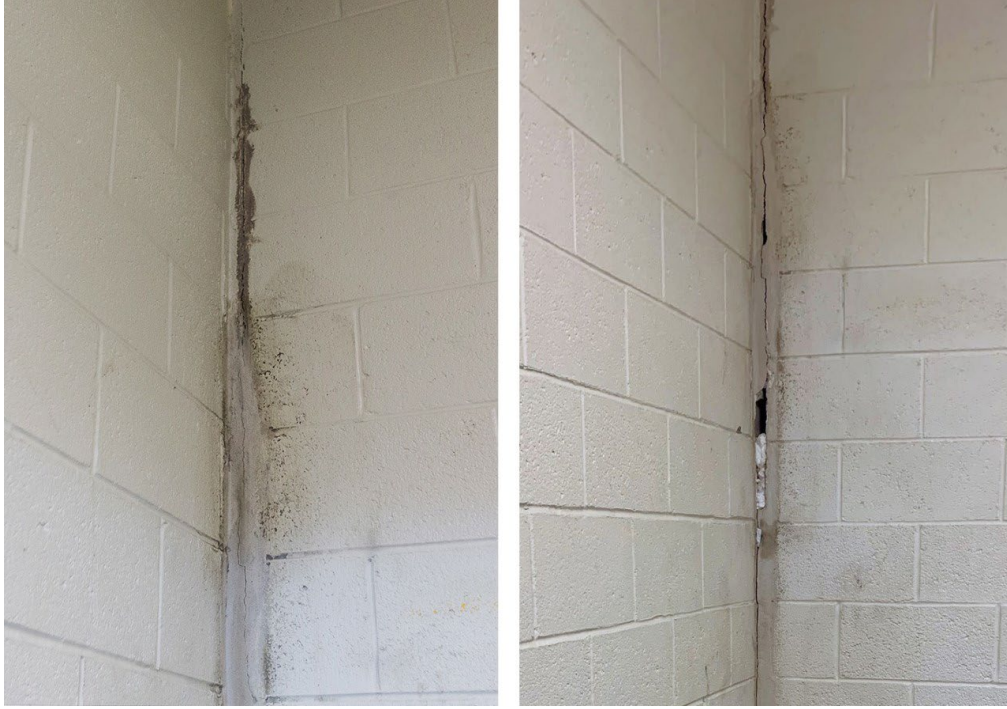
Figure 7: Crack in the Wall Between Adult and Juvenile Holding Cells Observed in 2015 (Left) and 2022 (Right)
