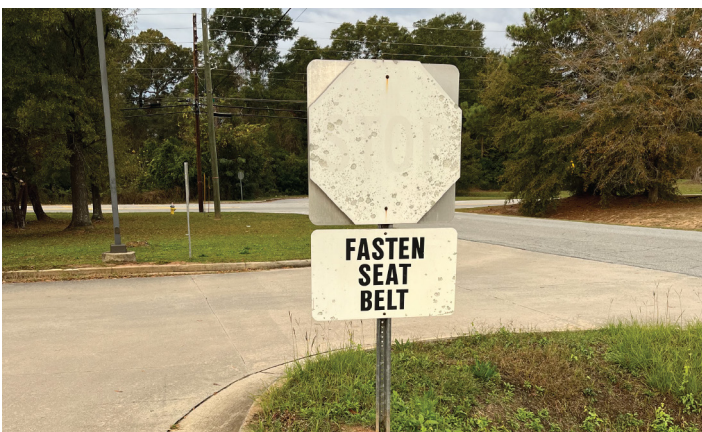
Figure 4. Example of Faded Stop Sign
