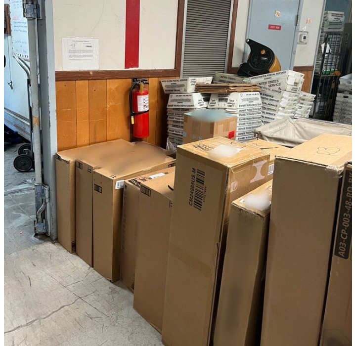
Blocked Electrical Panel
