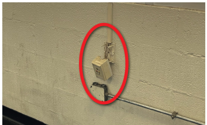
Figure 6. Broken Outlet in the Corryville Station Lobby
