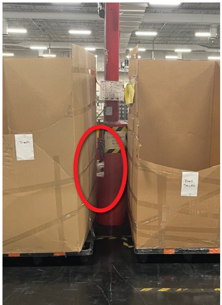
Figure 5. Blocked Fire Extinguisher at the Mid City Cincinnati Carrier Annex
