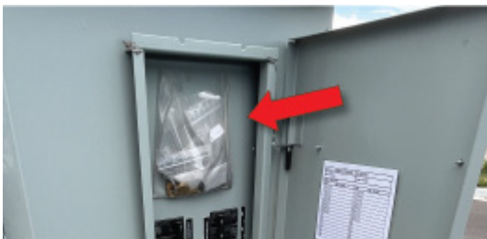
Figure 2. Electrical Panels Were Unlocked with Keys Inside
