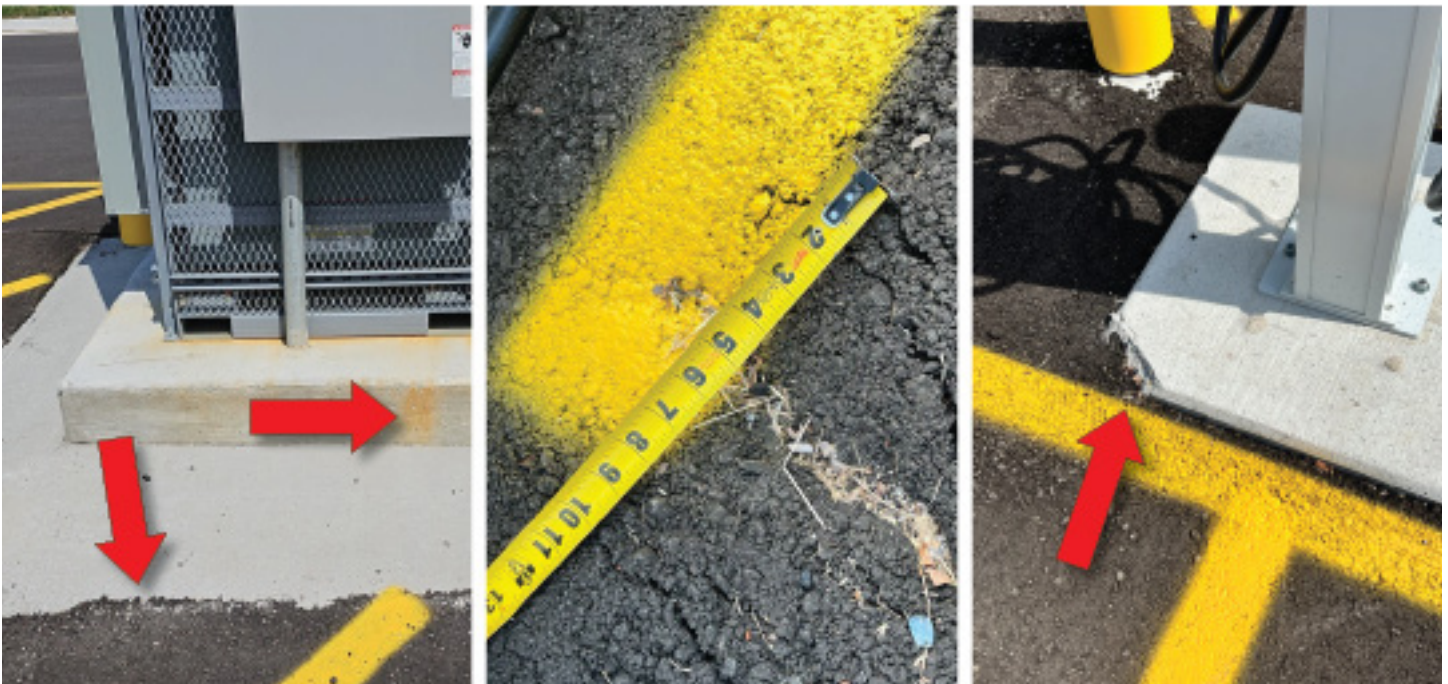
Figure 7. Rust, Chipped Concrete, and Sinking Asphalt in Parking Lot.
