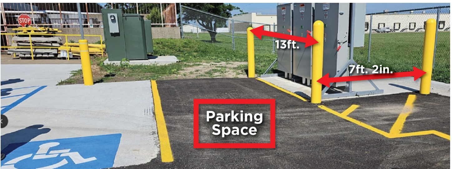
Figure 6. Insufficient Number of Bollards Near Electrical Panels
