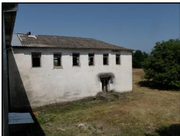
The roof of the Kuchatani school's attached gymnasium is made of asbestos-containing materials (photo by OIG).
