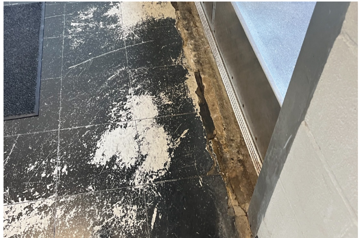
Chipped and Unleveled Floor Tile
