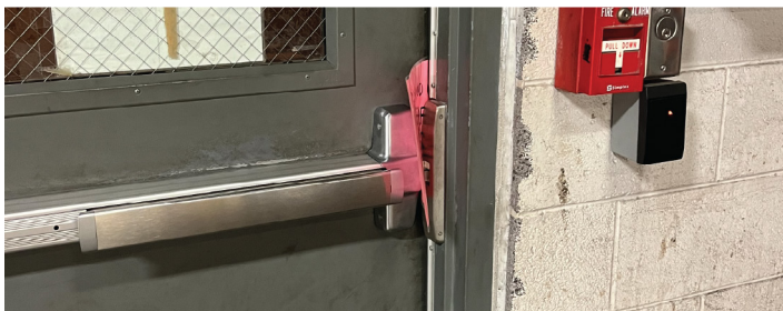
Figure 6. Laminated Paper to Prop Open Exit Door
