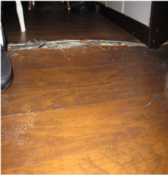
Picture 5 – Floors (non-HS): Property ID 6978; tears in basement flooring, partially covered with tape, tripping hazard.
