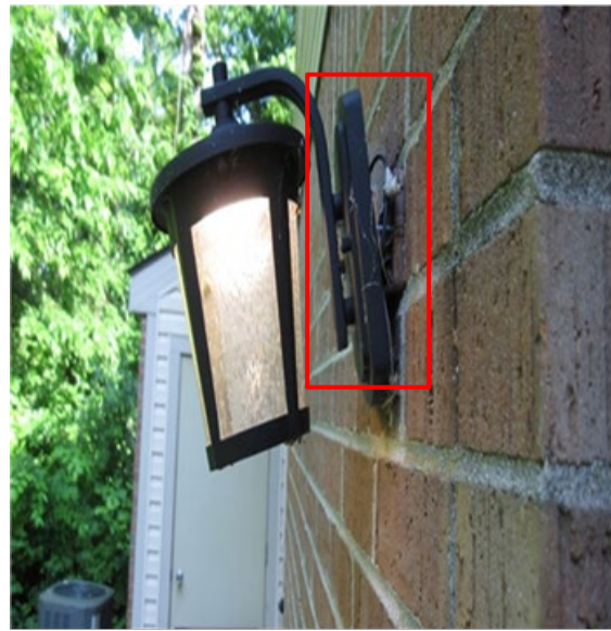
Picture 14 – Electrical (non-HS): Property ID 6438; exposed, frayed electrical wires on exterior light fixture, and light fixture is not secured.
