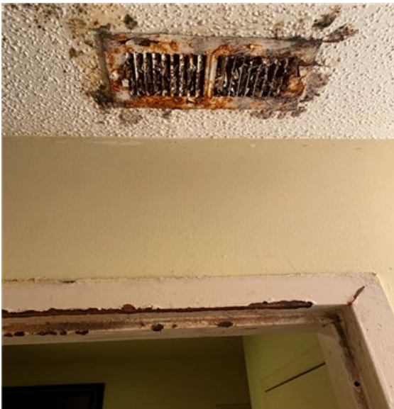
Picture 7 – Hazard (NLT): Property ID 3812; rusted ceiling vent in bathroom, water damage, and possible mold or mildew on ceiling.
