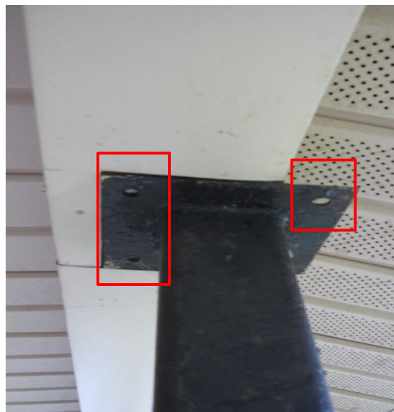
Picture 18 – Top of railing off center and missing all screws.
