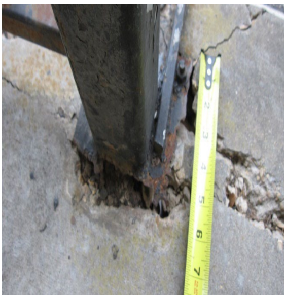
Picture 19 – Crumbling concrete with rusted base showing screws missing or not connected.
