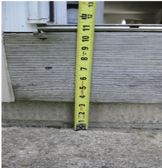
Picture 3 – Other hazard (NLT): Property ID 6978; high entryway step with approximate 11-inch rise, elderly occupant uses a walker, poses a falling hazard.
