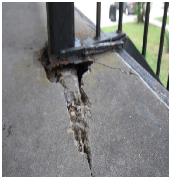
Picture 20 – Alternate view of base with missing and crumbling concrete showing missing screws.
