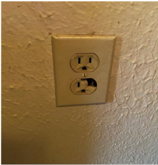
Picture 13 – Electrical (LT): Property ID 3812; broken outlet cover plate where electrical plug is inserted, in bedroom.
