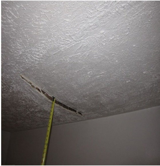
Picture 9 – Ceiling (non-HS): Property ID 2652; cracked and bulging ceiling above a child's bed.
