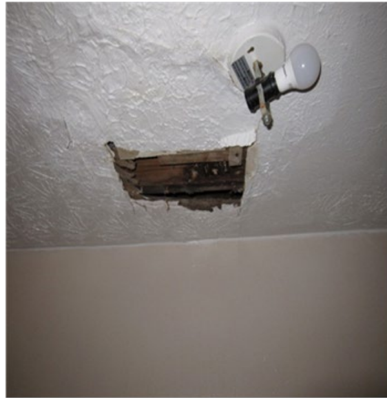
Picture 10 – Ceiling (non-HS): Property ID 1435; hole in kitchen ceiling.
