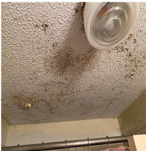
Picture 11 – Ceiling (non-HS): Property ID 3812; water stains, water damage, and possible mildew or mold on bathroom ceiling.
