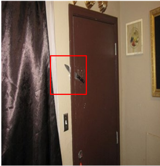
Picture 1 – Doors (NLT): Property ID 5129; damaged frame with knife wedged into doorframe for security.
