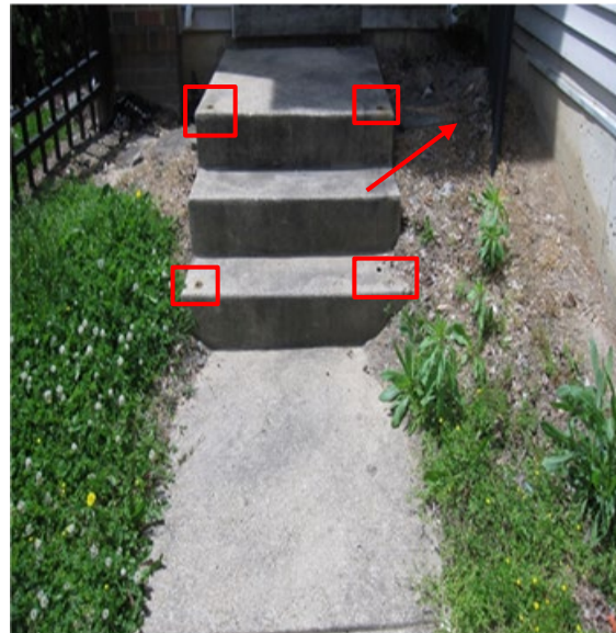
Picture 4 – Other hazard (NLT): Property ID 6978; railings not connected, set to the side, causing possible falling hazard on entry steps.
