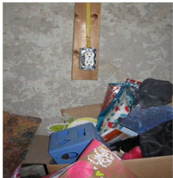
Picture 12 – Electrical (LT): Property ID 6978; missing outlet cover in basement, exposing interior of outlet box.
