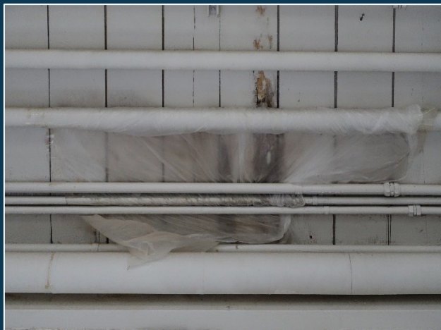
Evidence of water intrusion from the roof, with plastic covering a single-level housing unit ceiling during FCI Tallahassee inspection
