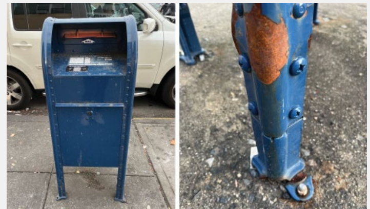
Blue collection box with missing bolts and corrosion seen in Queens, NY, during mail theft mitigation audit. Source: OIG photograph.
