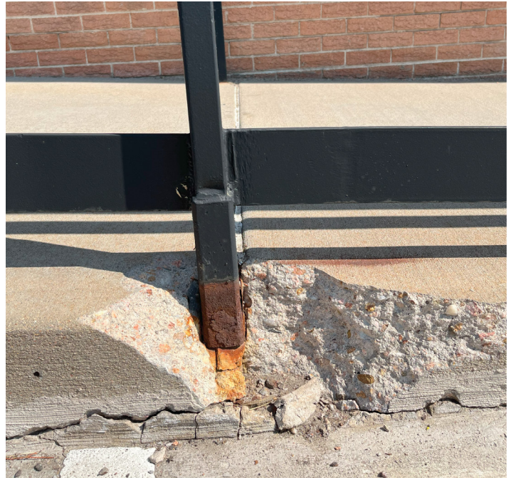
Figure 5. Loose Handrail
