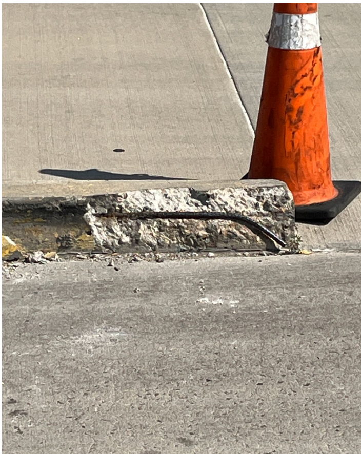
Figure 5. Concrete Bumper With Exposed Rebar at Dock Truck Bay
