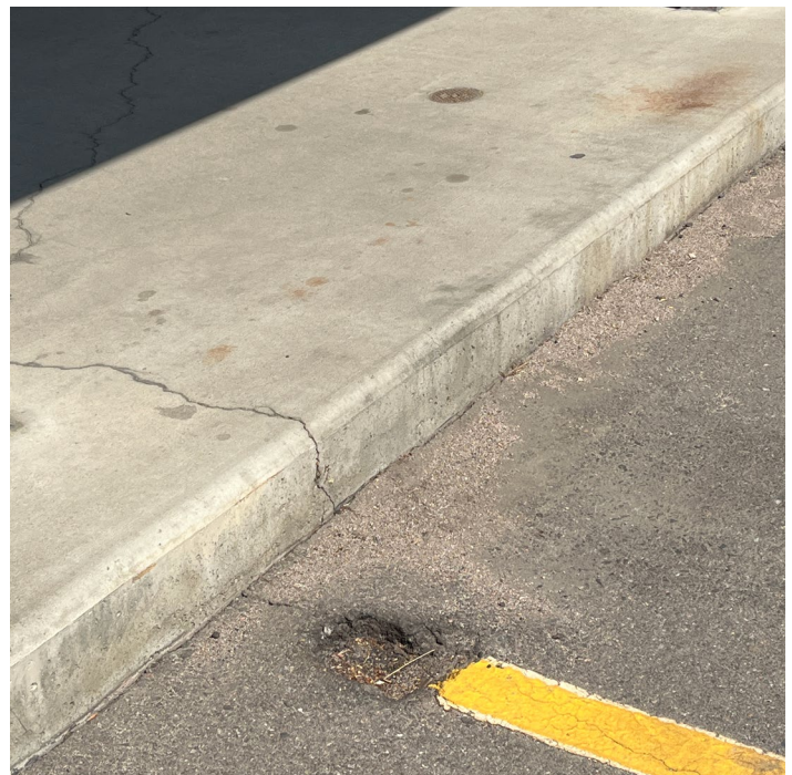
Figure 4. Concrete Bollard Not Installed at Carrier Loading Area
