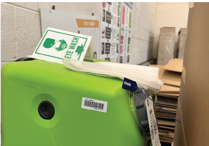
Figure 5. Blocked Eyewash Station
