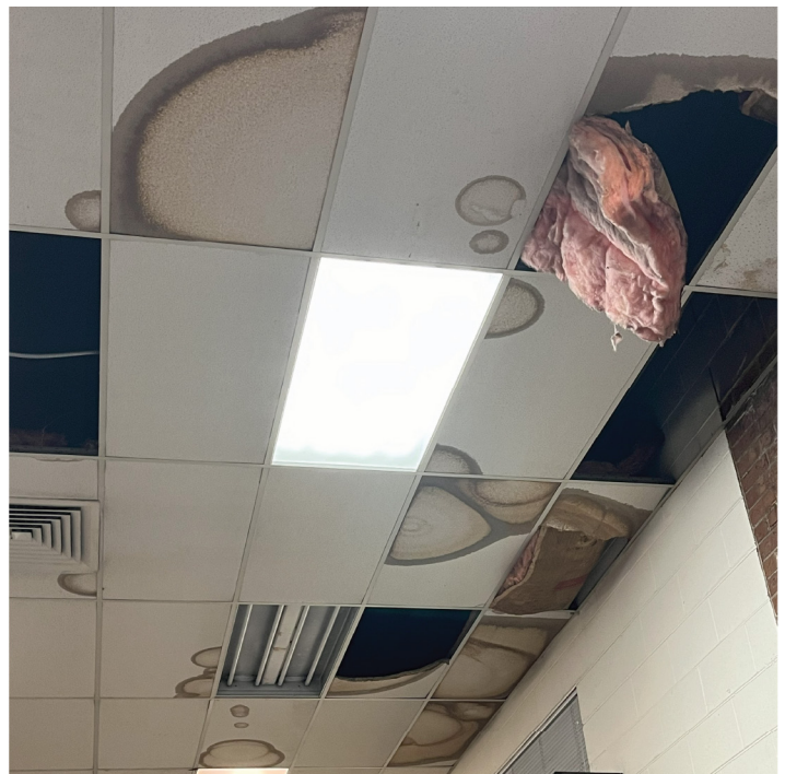
Figure 6. Missing and Stained Ceiling Tiles on the Workroom Floor
