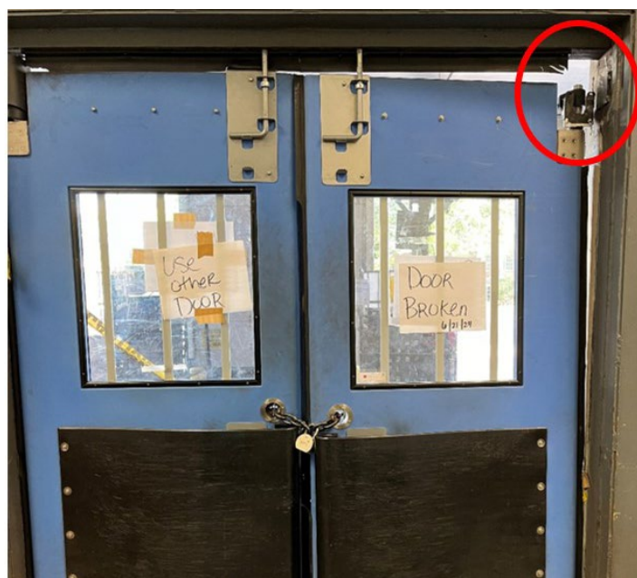
Figure 6. Broken Bolts on Back Door at Tuscaloosa MPO
