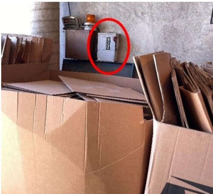
Figure 5. Blocked Circuit Box at Northport PO
