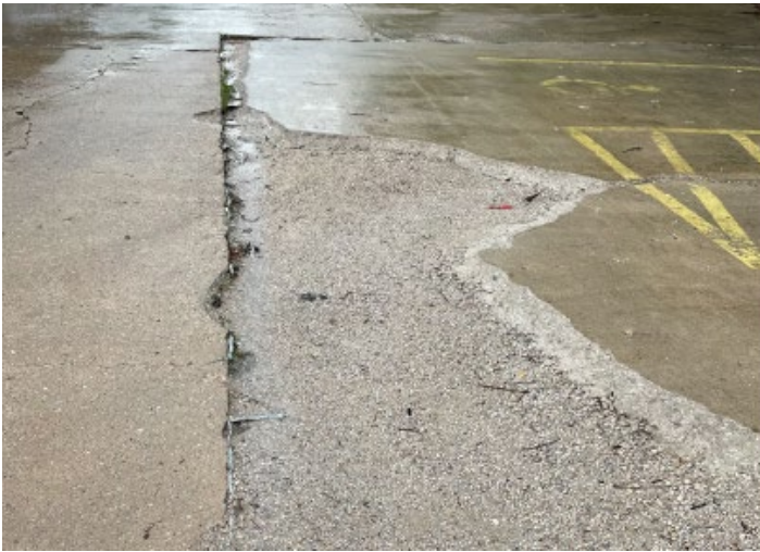
Figure 4. Concrete Cracks in Employee Parking Lot
