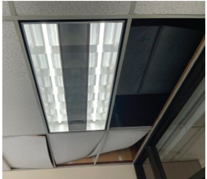
Figure 5. Missing Ceiling Tiles in Customer Lobby
