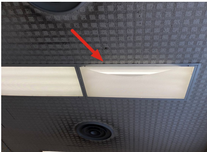
Figure 4. Light Cover Not Secure in Retail Lobby
