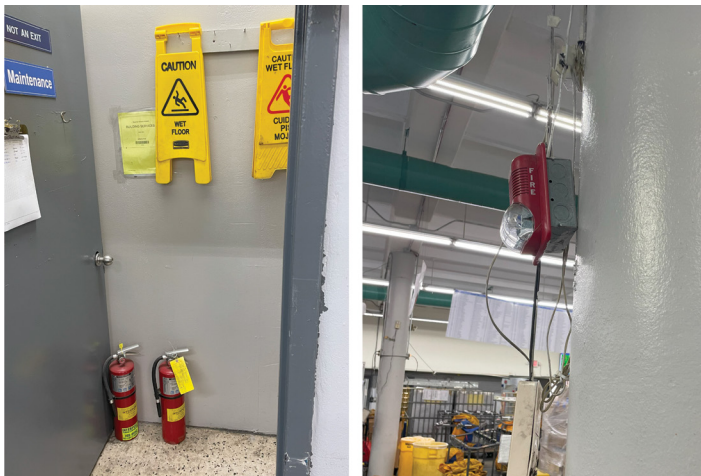
Figure 4. Unmounted Fire Extinguishers and Fire Alarm
