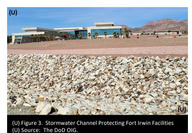
Fort Irwin's mission. Figure 3 shows an example of a rock stormwater channel built on Fort Irwin in front of facilities.
