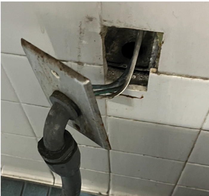
Figure 6. Loose Water Pipe Socket in Men's Restroom
