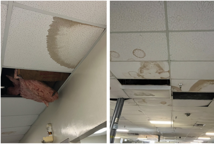
Figure 5. Stained and Missing Tile in Men's Restroom and Workroom Areas
