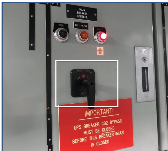
Figure 2. Unprotected circuit breaker at Hines Information Technology Center.
