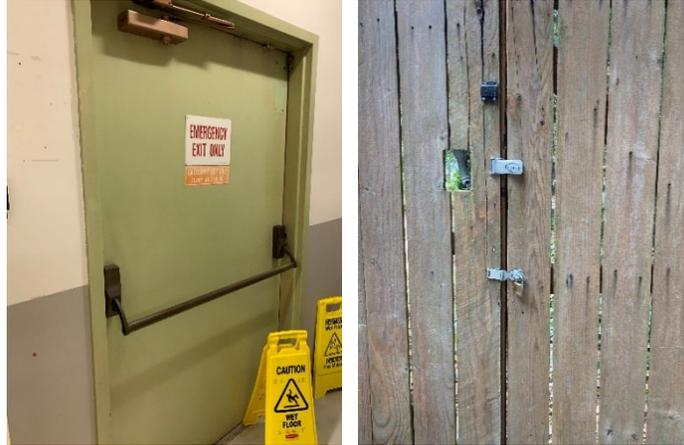
**Photograph 1 (left): Door marked as emergency exit led to patio with locked gate.
