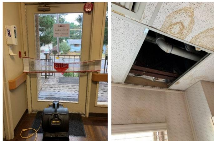
**Photograph 3 (left): Pathway to exit blocked by fan.
