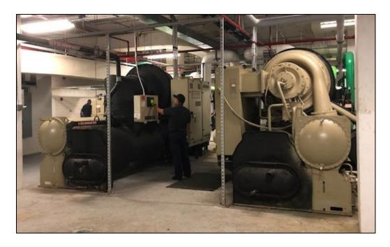
Chillers cool buildings by removing heat from a liquid coolant to cool and dehumidify the air. A breakdown in a chiller may lead to rising temperatures and humidity within the building and possible building closures.
