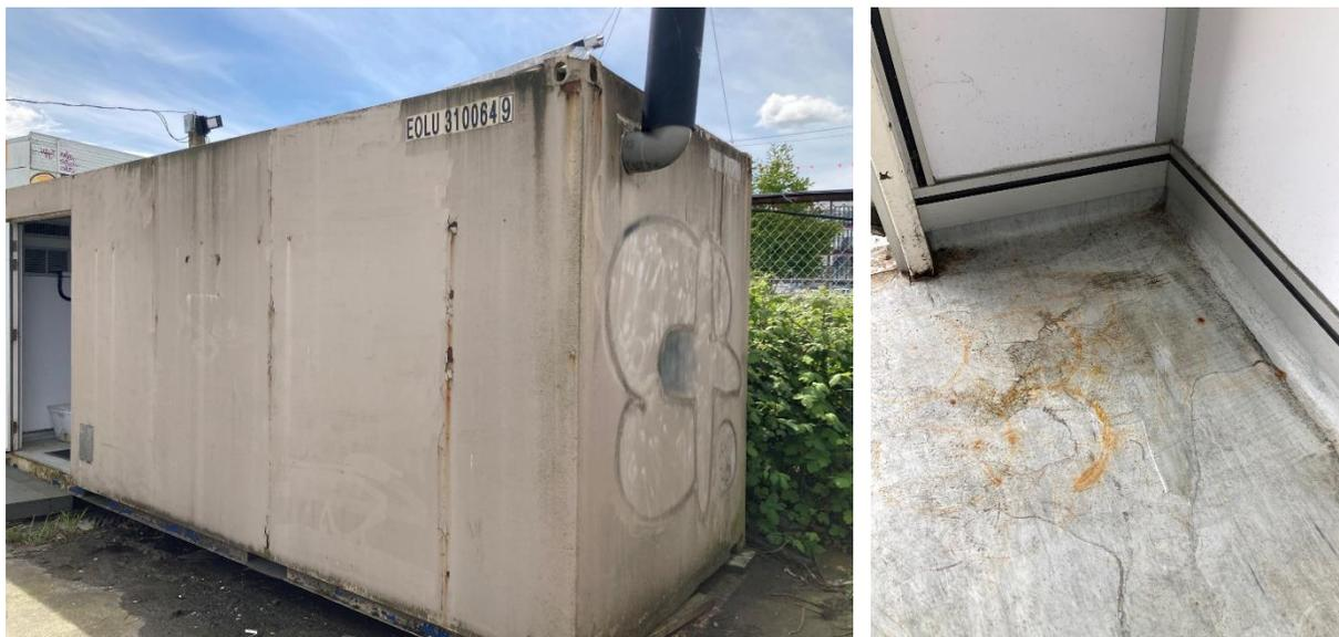
**Figures 3 and 4:** The exterior and interior conditions of Consulate General Vancouver's mail screening facility. (Source: Consulate General Vancouver.)
