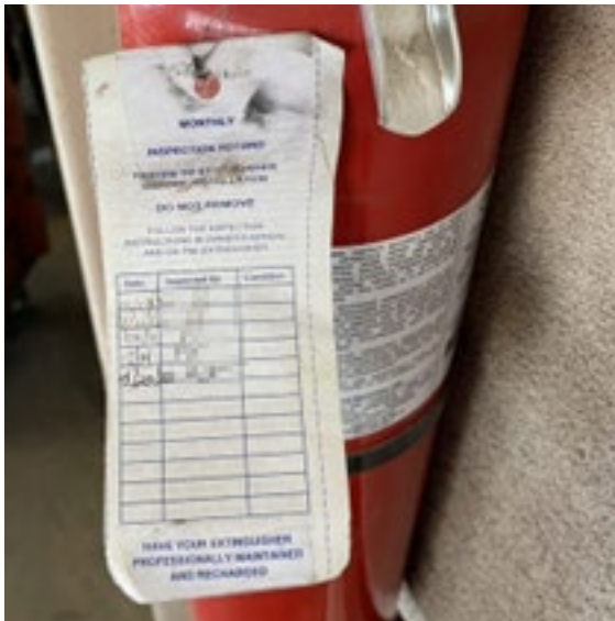
Figure 2. Fire Extinguisher not Inspected
