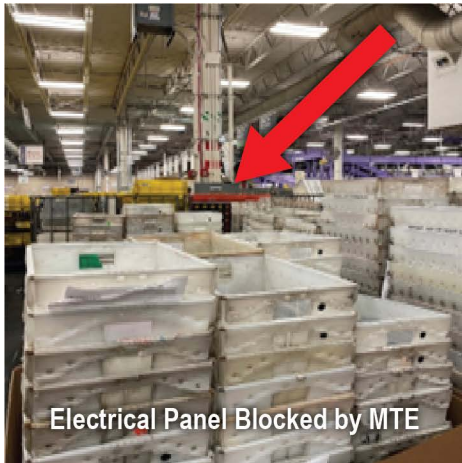
Figure 10. Blocked Electrical Panel and Fire Extinguisher
