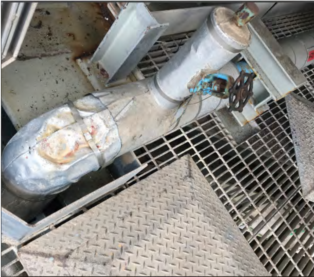
Figure 3: Degraded Insulation
