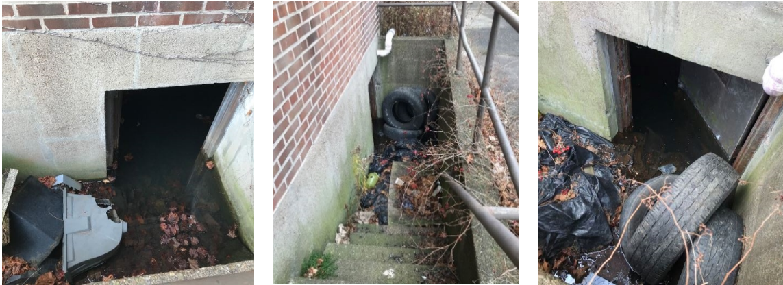
Examples of flooded stairwells with open doors leading into flooded crawlspaces
