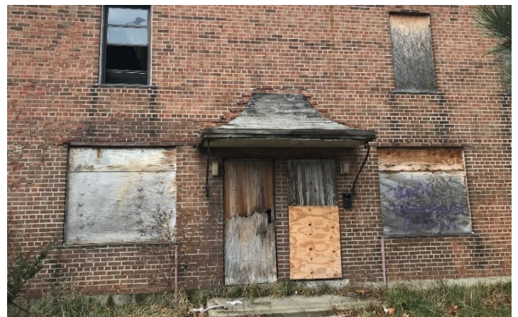
Deteriorated awning and open 2 nd floor window
