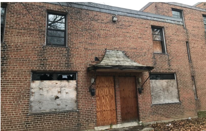
Deteriorated awning and broken glass on 1 st floor window
